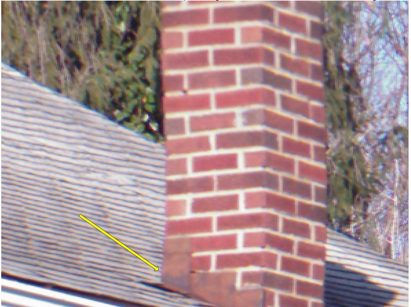
Saddle Flashing(s) Recommended
